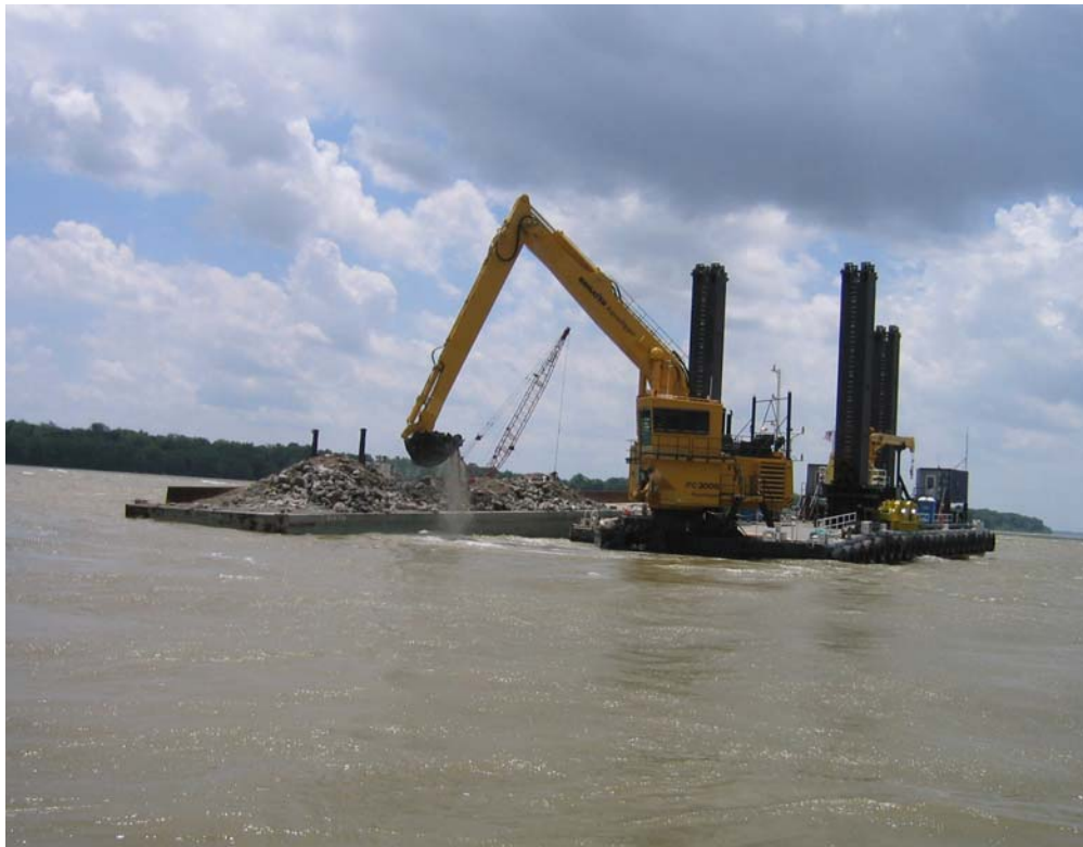
The excavator dredge OLM-033 at work on the Olmsted Dam project on the Ohio River.
