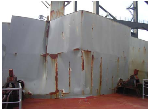
Ship Breakwater Damaged by Boarding Seas
