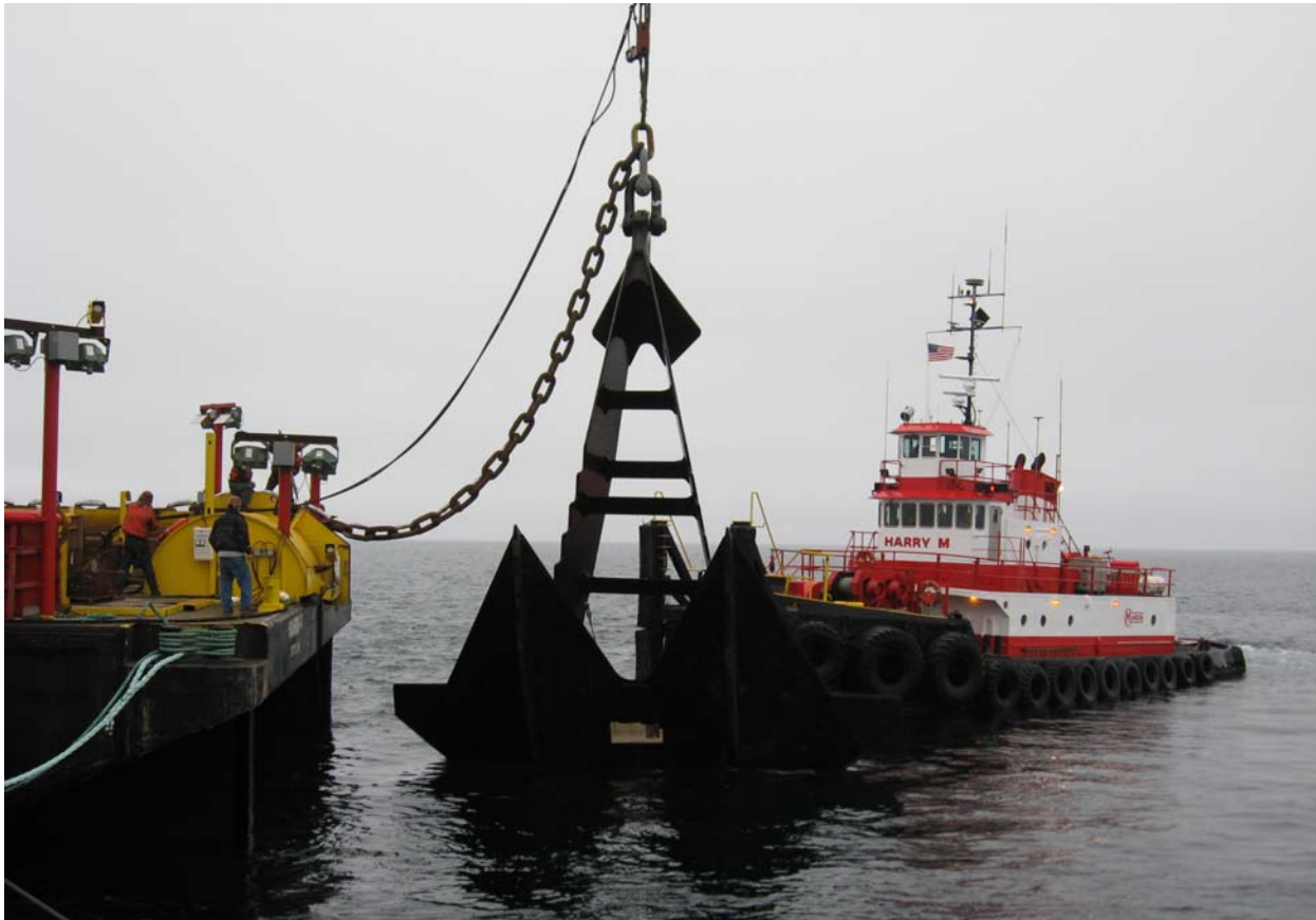
Setting one of the 60 tonne high performance anchors and 114 mm chain.
