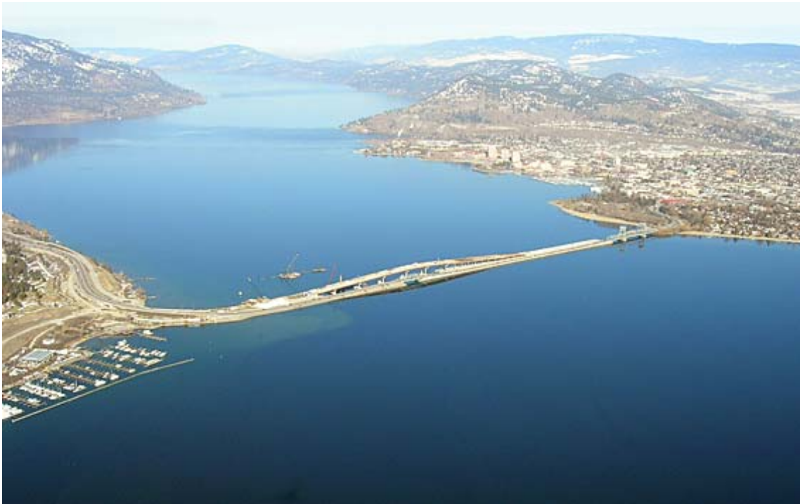
W.R. Bennett Bridge crosses Lake Okanagan at Kelowna B.C.
