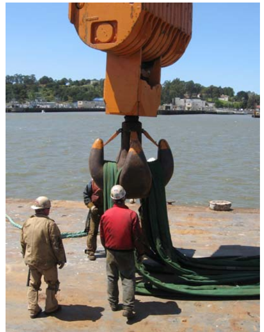
Shown above is the rigging for the load test.
