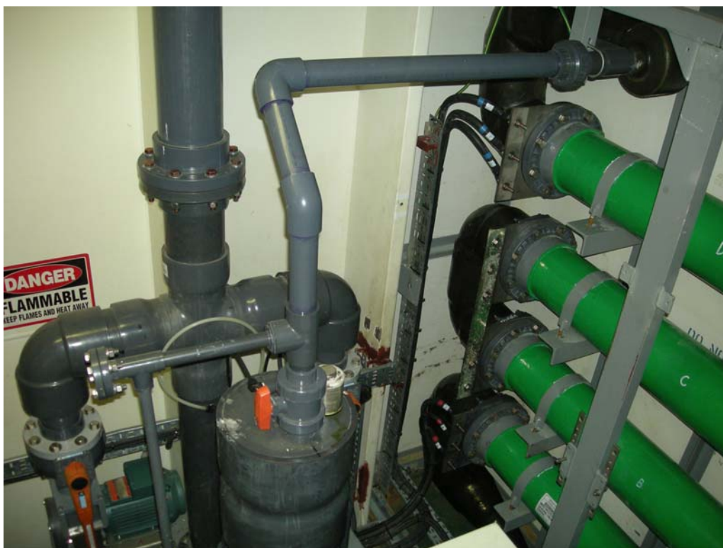
Figure 1. Ballast water treatment module on the S/R AMERICAN PROGRESS
